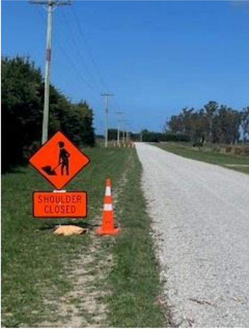
Figure 3 - Simple TTM set up for a quiet rural road
